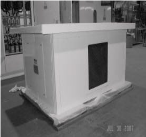
Enclosure for Generator Neutral Reactor Figure 3
